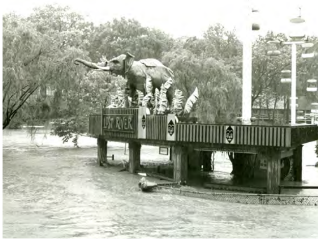
The entrance to the Lost River ride with water nearing the top of the fence, June 1972
