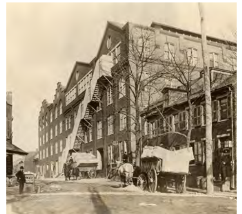
Photograph of the Lancaster Caramel Co. factory from the intersection of Church St. and S. Duke St., ca. 1896-1900.
